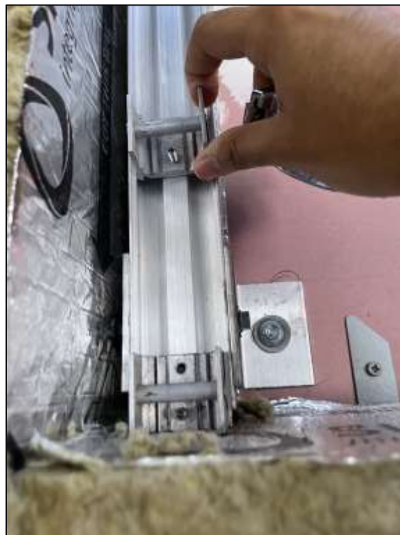
Picture 6: Panel holding clamps supported onto the runners.
