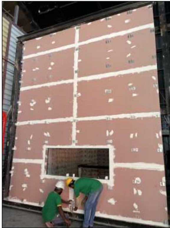
Picture 1: View of the wall brackets fixed onto the base wall.
