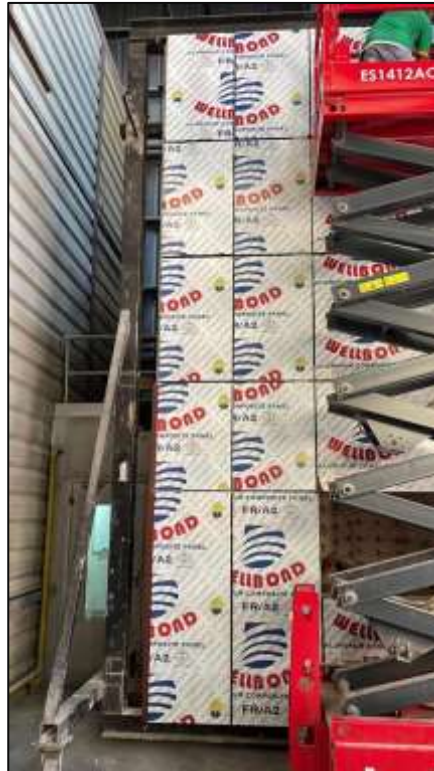
Picture 11: View of installing the cladding panels.
