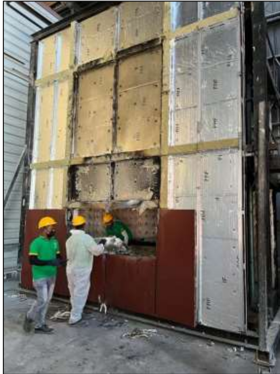
Picture 21: Dismantling view.
