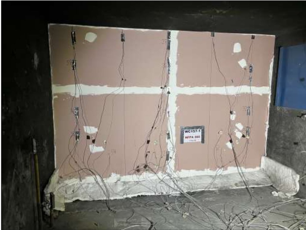
Picture 21: The interior of the base wall in the second-floor test room at the end of the test.
