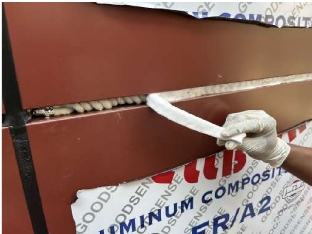
Picture 10: Ceramic piece being inserted into the panel joints after fixing the spiral threaded backers.
