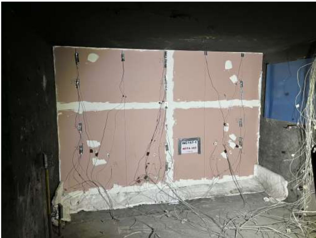
Picture 14: The interior of the base wall in the second-floor test room at the beginning of the test.
