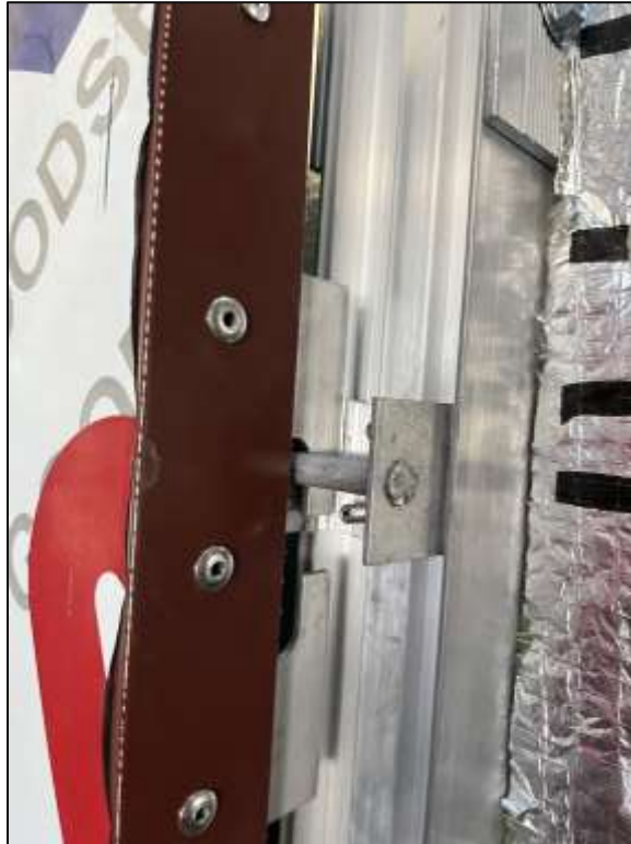
Picture 9: Method of fixing the panel in place with the support of panel clamps.
