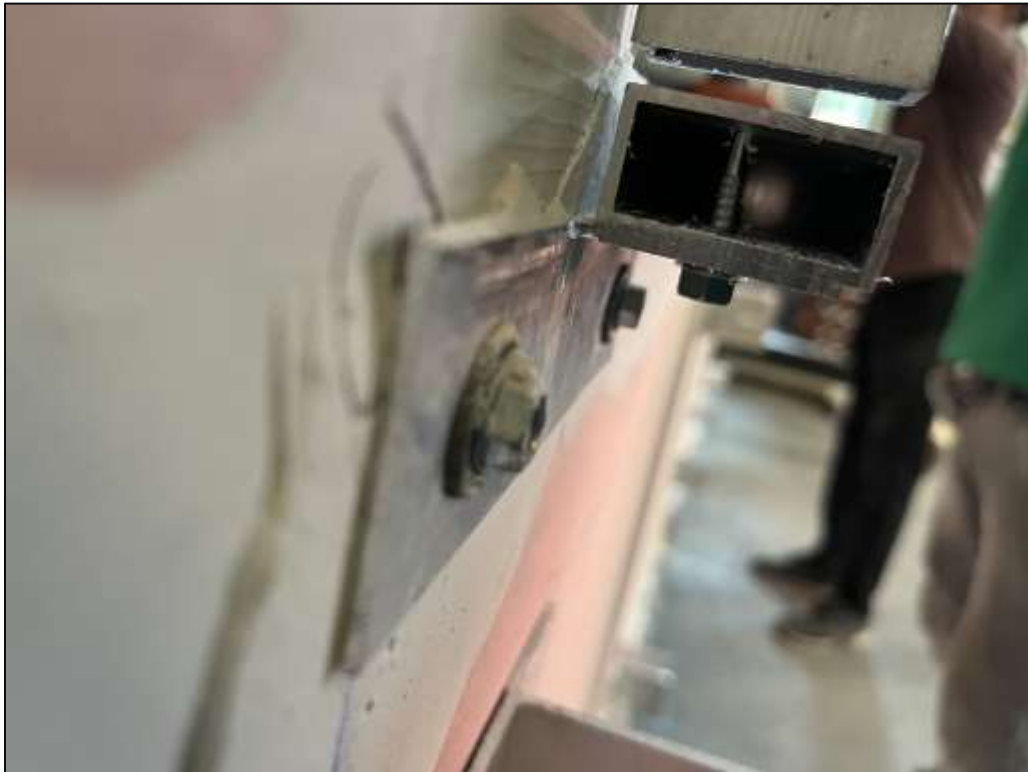
Picture 3: A close-up side view of the window perimeter tube channel.
