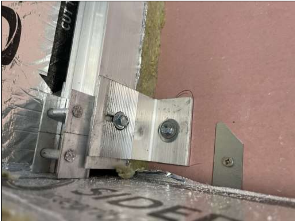
Picture 5: View of the runner to wall bracket fixing method.
